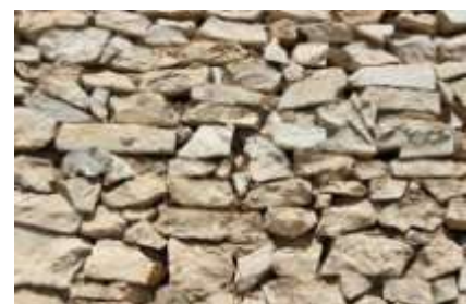
Detail of quartz sandstone bricks in War Memorial Tower
