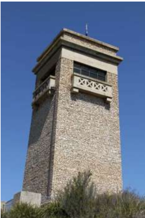
Goulburn War Memorial Tower
