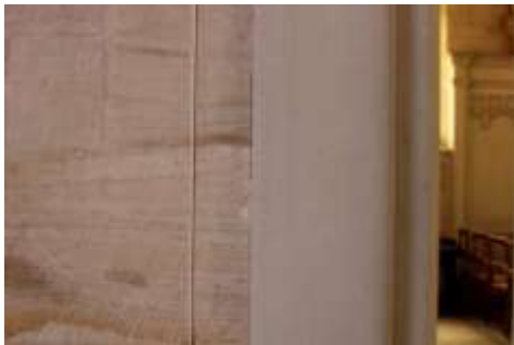
Edge of Screen (Bundanoon Sandstone) that separates the Memorial Chapel from the northern aisle. The screen abuts the coarser golden Marulan Sandstone. The Chapel is entirely constructed of Bundanoon Sandstone.
